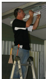
Graham installing the lighting
